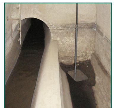
FLOW MEASUREMENT IN NARROW UNDERGROUND U-SHAPED CHANNEL
