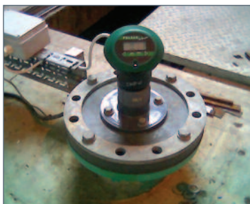
IMP ON A LIQUID LIME TANK
