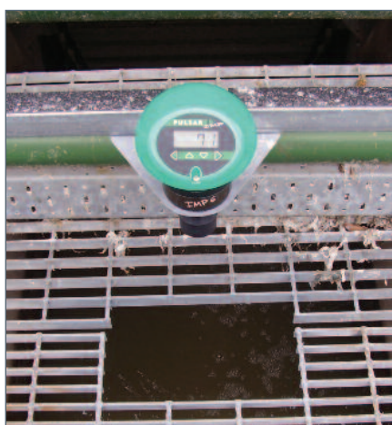
IMP CONTROLLING GATE HEIGHT
