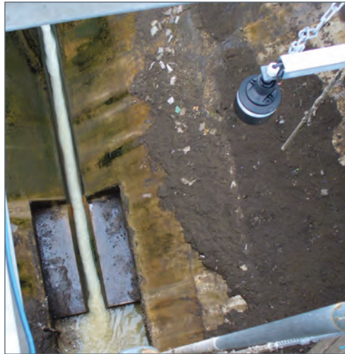
WET WELL 6m WITH LADDER AND FLOAT
