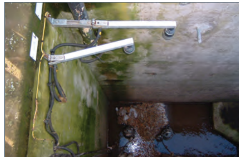
HINGED BRACKET OVER A WET WELL
